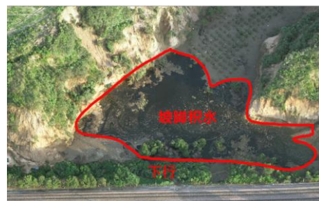
图2 铁路水害沿线某路堤坡脚积水航拍图 Fig.2 Aerial photo of rainfall accumulation at the foot of an embankment along water damaged railway
